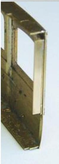
The non-window end though is a single thickness of etch. As you can see, I added some strengthening angle strip in the corners, which will be invisible through the opaque lavatory windows at this end.
